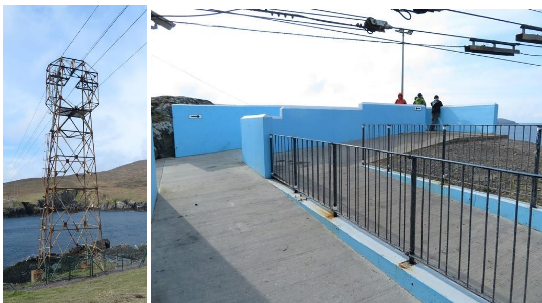
Plate 15.2 Mainland-side pylon (left) and landing platform (right).
