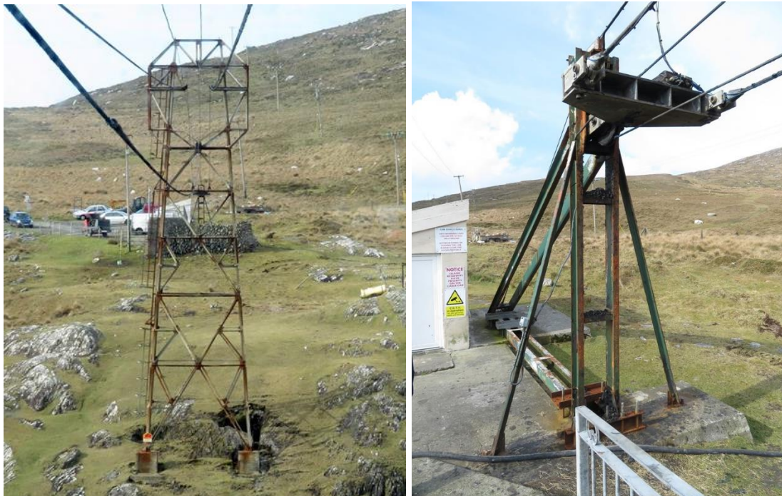
Plate 15.6 Island-side pylon (left) and anchor point (right).
