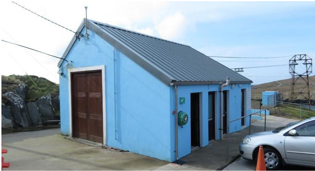
Plate 15.3 Mainland-side line station building
