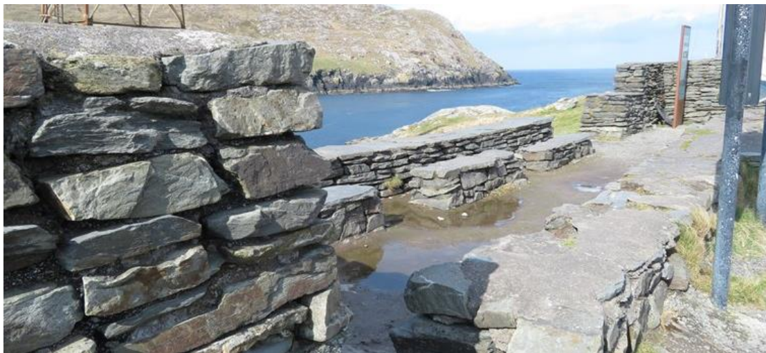
Plate 15.4 Stone walls and benches on the mainland side of the site
